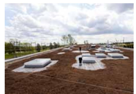
Installed system substrate "Rockery Type Plants".
