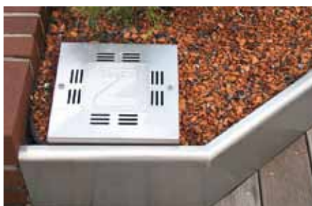
An inspection chamber incorporated into the system build-up
