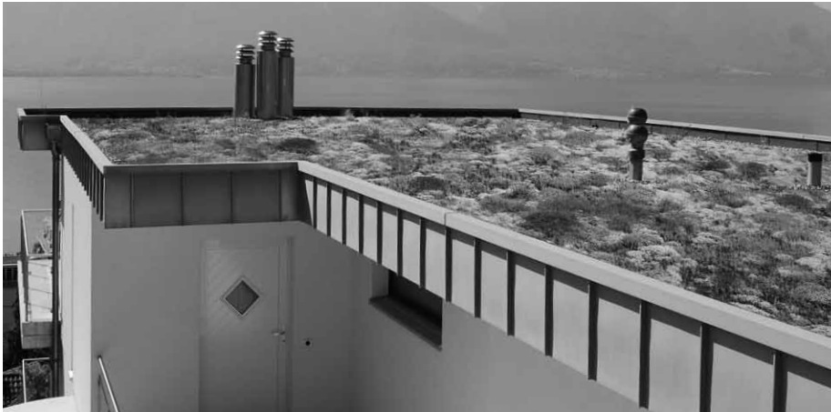
Extensive Green Roof
