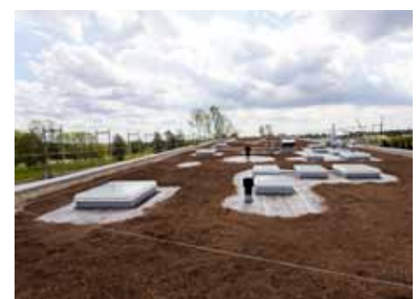
Installed system substrate "Rockery Type Plants".
