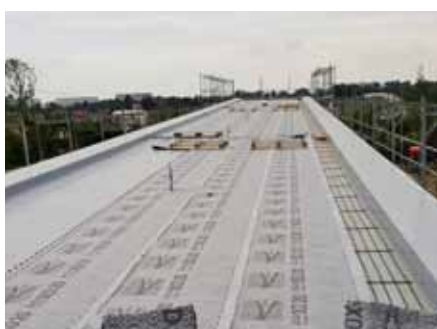
The System Build-up "Rockery Type Plants" provides the foundation, this is the drainage element Fixodrain® XD 20.
