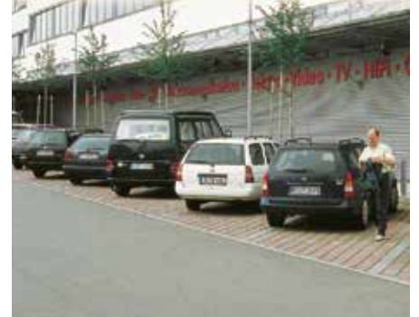
Fire brigade accessible asphalt surface.
