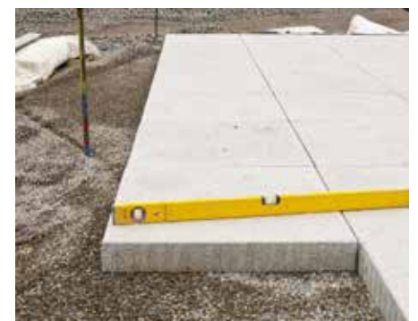
After the Filter Sheet TG is rolled out over the drainage layer, the bedding layer ist levelled to provide adequate stability to the overlying slabs.
