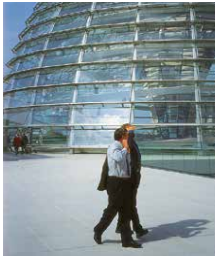
The combined protection and drainage layer, which has been applied here still protects the waterproofing membrane under the large scale concrete slabs .
