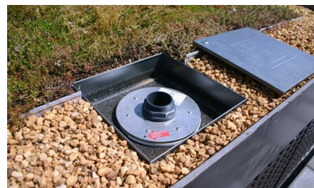
The Run-off Limiter Set is installed above the roof drain.
