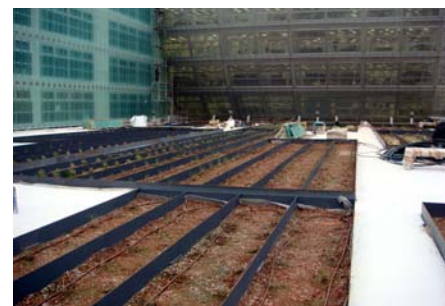
To make sure the vegetation maintains its green character even during hot summer months dripper lines have been installed within the planting beds.
