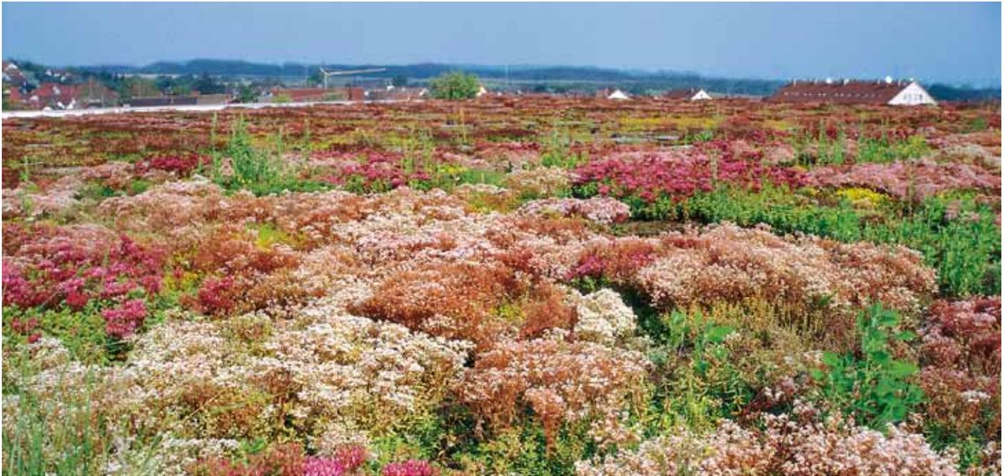
The "Sedum Carpet" is a standard build-up for extensive Green Roofs. It is a shallow and lightweight Green Roof type with an attractive "back-to-nature" appearance, that requires little maintenance.
