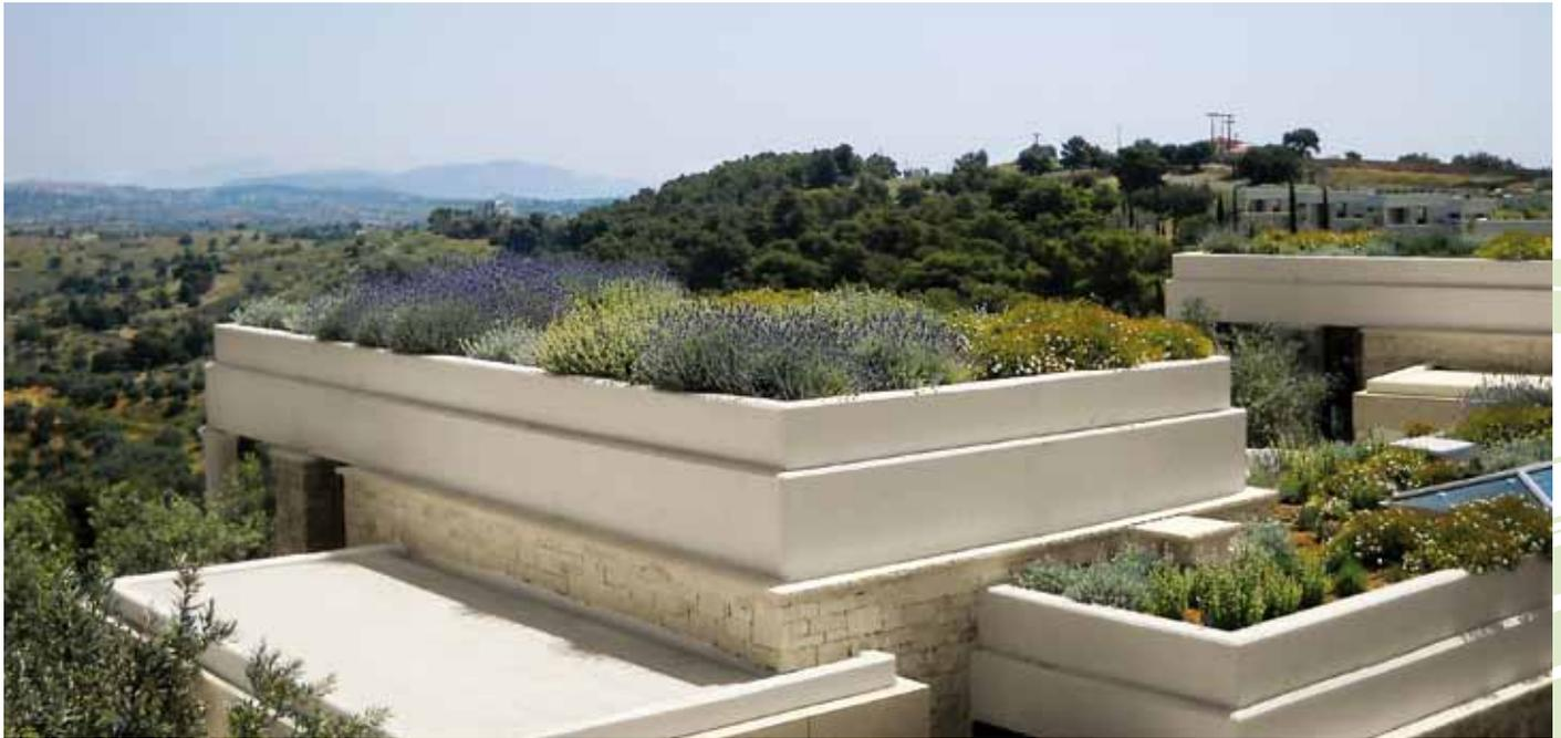
The semi-intensive system build-up “Heather with Lavender” allows for sophisticated planting design. Nevertheless, compared to intensive green roof build-ups, it manages with relatively low maintenance and relatively low build-up heights.
