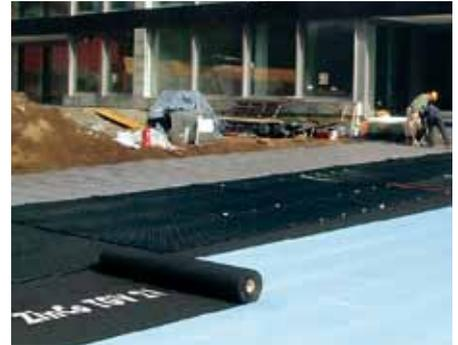
The characteristic of an inverted roof is that the insulation is above the waterproofing. The extruded polystyrene insulation (XPS) which is used for this kind of roof is impervious to water, but not to water vapour. Forming a vapour barrier directly above it when installing a Green Roof must therefore be avoided. Layers that prevent moisture from diffusing out mustn't be installed over the thermal insulating XPS boards and the layer above should be vapour permeable.
