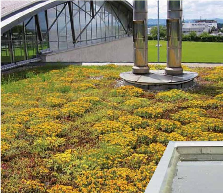
On 0°-roofs where deeper puddles might remain, the standard extensive system build-up is to be modified.
