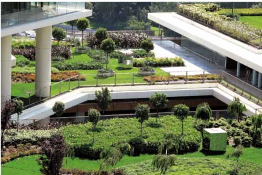
Intensive Green Roofs can most easily be compared to building a garden on a roof. They are usually multifunctional and accessible. They require more weight and a deeper system build-up. The maintenance is regular and depends on
