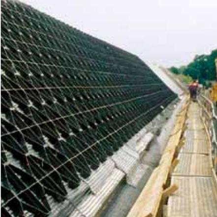
The system build-up "Steep Pitched Green Roof", based on the Georaster® elements, enables the installation of Green Roofs with slopes exceeding 20° and up to 35°. Above 35° special solutions can be designed by the ZinCo engineers.
