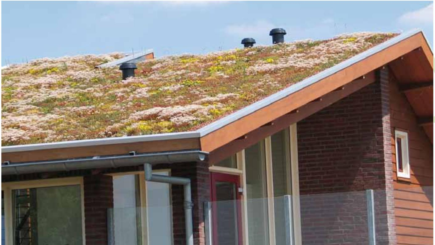
In general, flat roofs should have a slope of at least 2 %. Pitched roofs, as described in this brochure, start with a slope of 10° (18 %). From 10° on, the Green Roof system build-up differs significantly from system build-ups below 10°. Shear forces increase with the roof slope and have to be transferred into stable beams. The substrate layer has to be protected against erosion.
