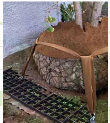
The tree anchorage system Robafix® is developed specially for root ball anchoring on intensive Green Roofs and underground car parks.
