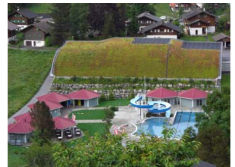
The collectors for warm water can be seen at the top right of the extensive green roof.
