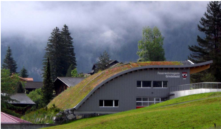
The Grindelwald fire station merges beautifully with the surrounding mountainside.
