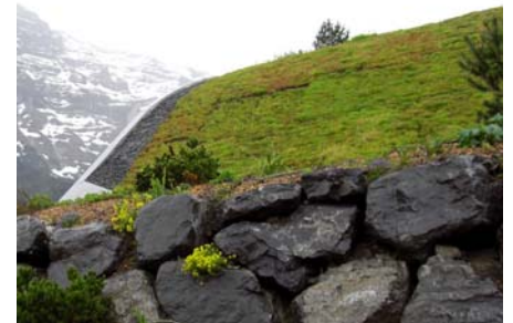
The sloped roof with newly-installed pre-cultivated vegetation mats.
