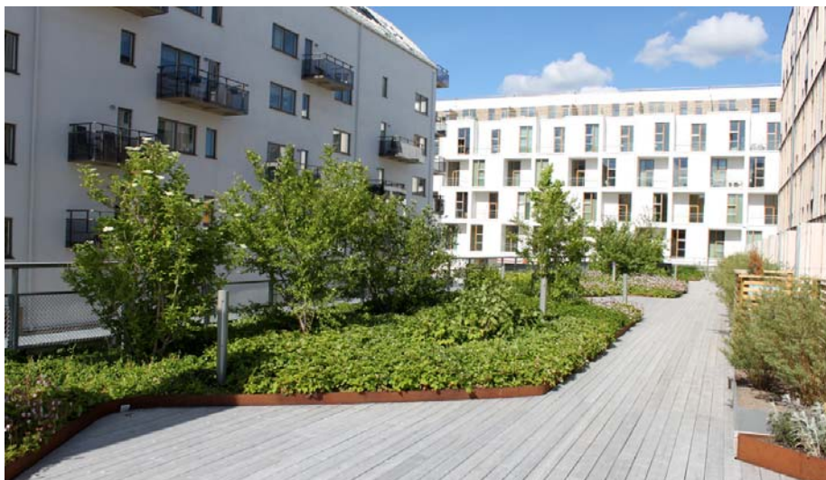
Corten steel boundaries separate the soft shapes of the planting areas from the wooden deck.
