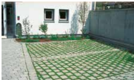
Pavement joint greening
