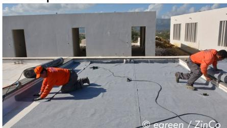
The protection mat TSM 32 is the first layer to be installed with an overlap on the root resistant waterproofing.
