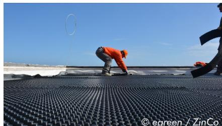
The Floradrain® FD 25-E drainage and water storage elements regulate the water balance in the System Build-up.
