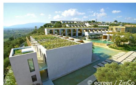
The green roofs protect the waterproofing membrane and provide a cooling effect in summer as they are like an additional layer of insulation.
