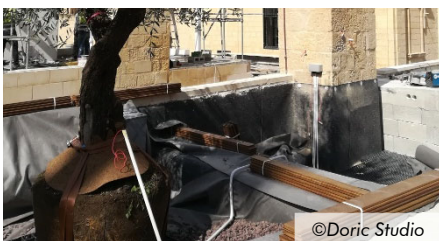
With the tree anchor system Robafix®, the tensioning straps are attached to three anchor points of the grid element, thus permanently securing the root ball.
