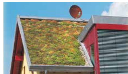
With this roof, which has a pitch of approx. 30°, a shear barrier was installed within the roof area, in addition to the stable eaves upstand.
