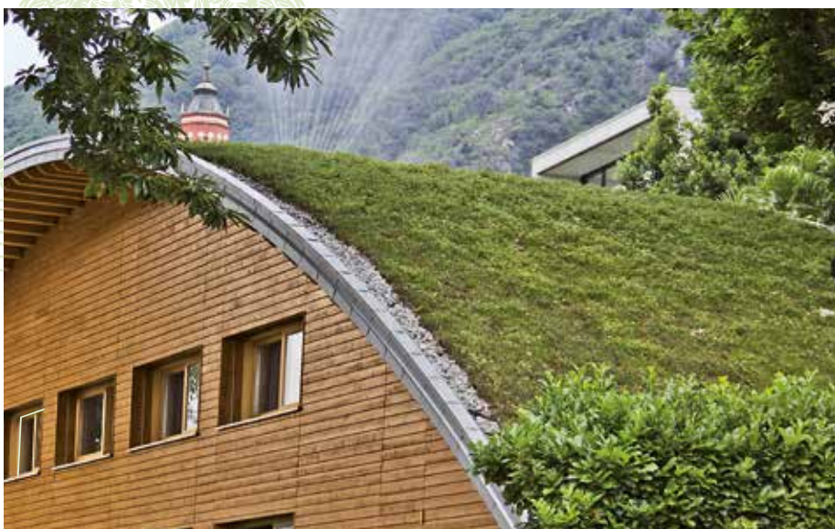
Pitched roofs require special measures to safeguard the vegetation.
