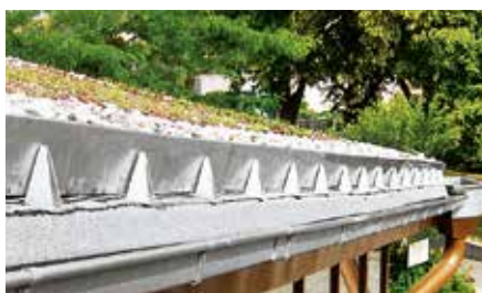
When determining the dimensions for eaves upstands or shear barriers, it is not only the saturated weight of the green roof build up that is relevant. Local snow loads must also be taken into consideration.
