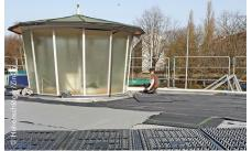
The drainage and water storage element Floradrain<sup>®</sup> FD 25-E was laid fully surfaced. Additional Solar Base Plates SB 200 were placed in the areas under the solar system.
