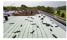
For another roof area, the rolled drainage mat Fixodrain® XD 20 with Aquafleece was chosen – here: subsurface irrigation with dripperlines.
