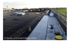
One part of the roof was covered with the water distribution, retention and drainage element Aquatec® AT 45 plus dripperlines.
