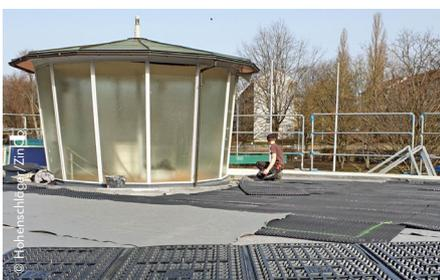
The drainage and water storage element Floradrain® FD 25-E was laid fully surfaced. Additional Solar Base Plates SB 200 were placed in the areas under the solar system.
