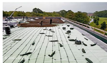
For another roof area, the rolled drainage mat Fixodrain® XD 20 with Aquafleece was chosen – here: subsurface irrigation with dripperlines.
