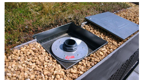
The Run-off Limiter Set is installed above the roof drain.
