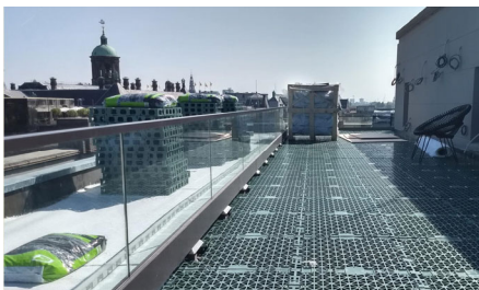
The RSX 65 spacer elements are placed on top of the Protection Mat SSM 45.
