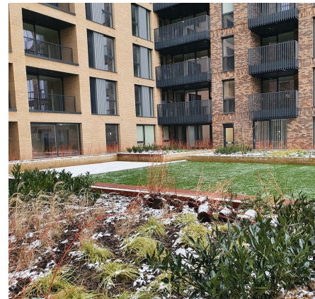
One of the podium decks during winter time shortly after installation.
