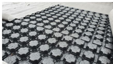
RS 60 retention spacers were used on all green roofs providing retention space below the wildflower/sedum build-up.
