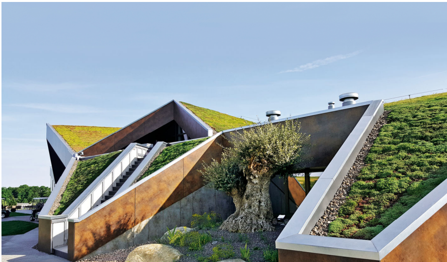
The roof of the new golf clubhouse building consists of different partial shapes with different inclinations.
