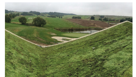
The approx. 2 m 2 vegetation mats were laid tightly joined without overlap.
