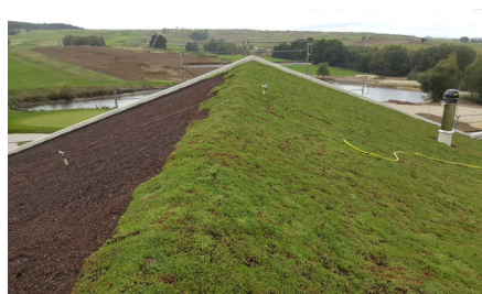
Pre-cultivated Sedum mats were used to achieve a quick ground coverage.
