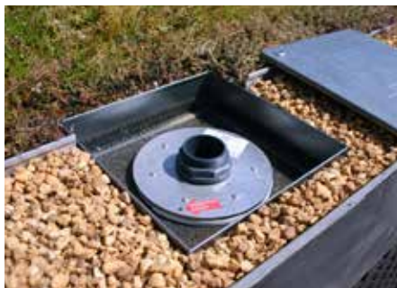
The limiter element is protected beneath the inspection chamber and regulates the slow discharge of water. At the same time, it acts as an overflow.
