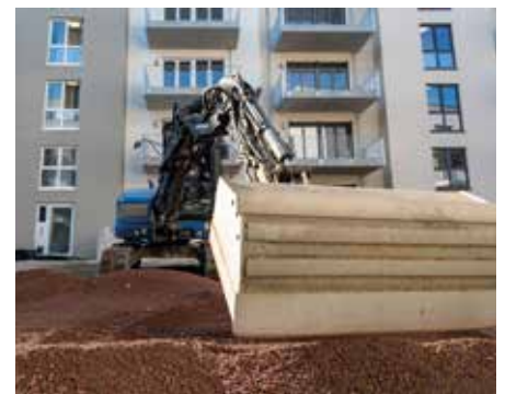
Thanks to the stable ZinCo system build-up with RSX 80, using diggers to apply the substrate is not a problem. © Strassen- und Tiefbau Urban GmbH
