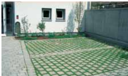
Pavement joint greening
