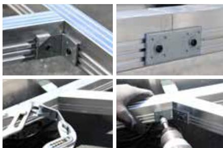
The various rail connectors allow for easy and stable assembly of the overall sub-structure.
