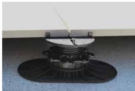
Given the slight pre-stressing already applied to the base plate during manufacture, solid support without wobbling is ensured right from the start. As a result, the pedestals are also stable and secure when the flooring and the additional weight are applied.
