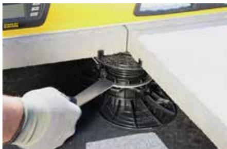
The new adjusting tool allows for the easy and subsequent adjustment and accurate setting of the required height, even after the pavers have been laid.
