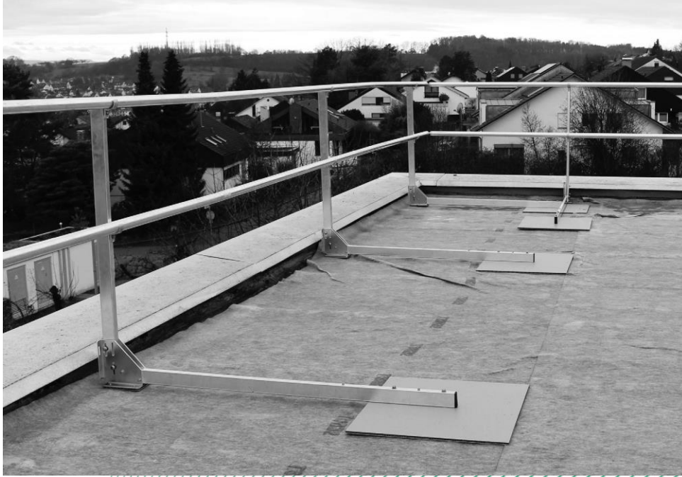
Fig. 1: Edge-protection system, type Fallnet® ASG
