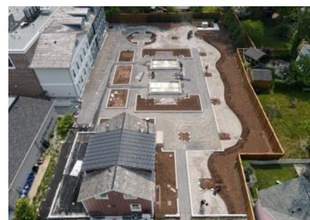
The roof area under construction shortly before laying the terrace slabs and planting.
