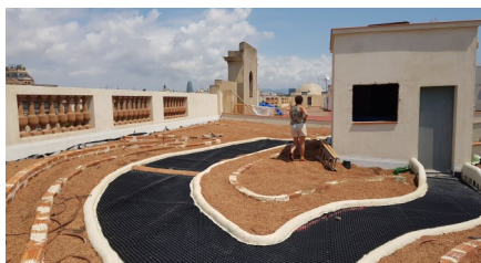
Both the ZinCo roof garden substrate made from recycled crushed clay tiles and the lime mortar for the boundaries are sustainable and natural products.
