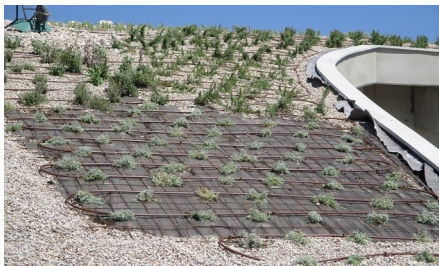
Good irrigation is important during the vulnerable growth phase after the initial planting in 2017. In steeper roof areas, the driplines are attached to separate lattices.
