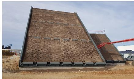
The system substrate Roof Garden is held firmly in place in the 100 mm high Georaster® elements.
