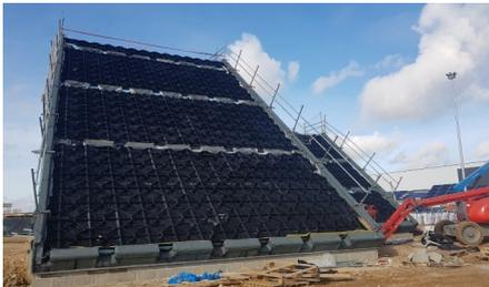
The 40–45° pitched steep roof areas are very well prepared with the system build-up Steep Pitched Green Roof with Georaster® elements
