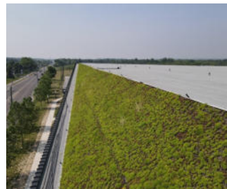
The steep pitched areas were realized with Georaster® elements.
