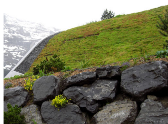
The sloped roof with newly-installed pre-cultivated vegetation mats.
