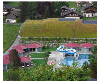
The collectors for warm water can be seen at the top right of the extensive green roof.
