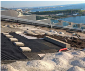
Protectodrain® and Elastodrain® mats ensure the safe drainage of exceeding water on the entire surface.
