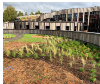
The substrate is applied in different heights to allow for a wide range of plants to thrive.
