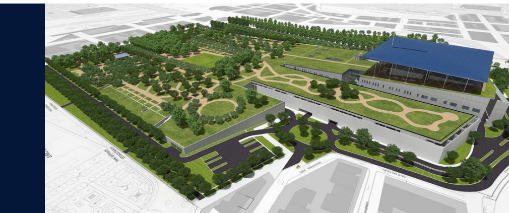
The roof of the opera is covered with a ca. 10,000 m 2 large solar plant.
