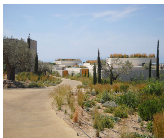
The roofs were predominantly planted with aromatic herbs and small shrubs, but also with grasses which are typical for this region and can cope with the heat very well.
