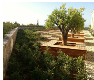
The room for root development of the olive trees was extended by special planting troughs.
