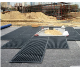
Stabilodrain® elements applied on the approximately 15,000 m 2 of ceiling surface of the underground parking provide a stable base for green areas, paths and seating.
