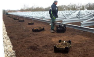
The Sedum plug plants are planted on the roof.
