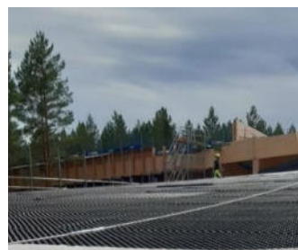
The System Build-up with Floradrain® FD 40-E was chosen. It's an optimal basis for a green roof with a high level of species diversity.
