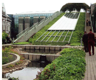
Over stairs on both sides of the pitched green roof you get on the main roof garden.
